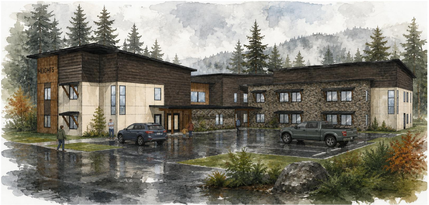
Eklund at Gales – 24-unit multi-family new construction
