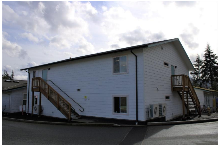
Exterior of shelter expansion
